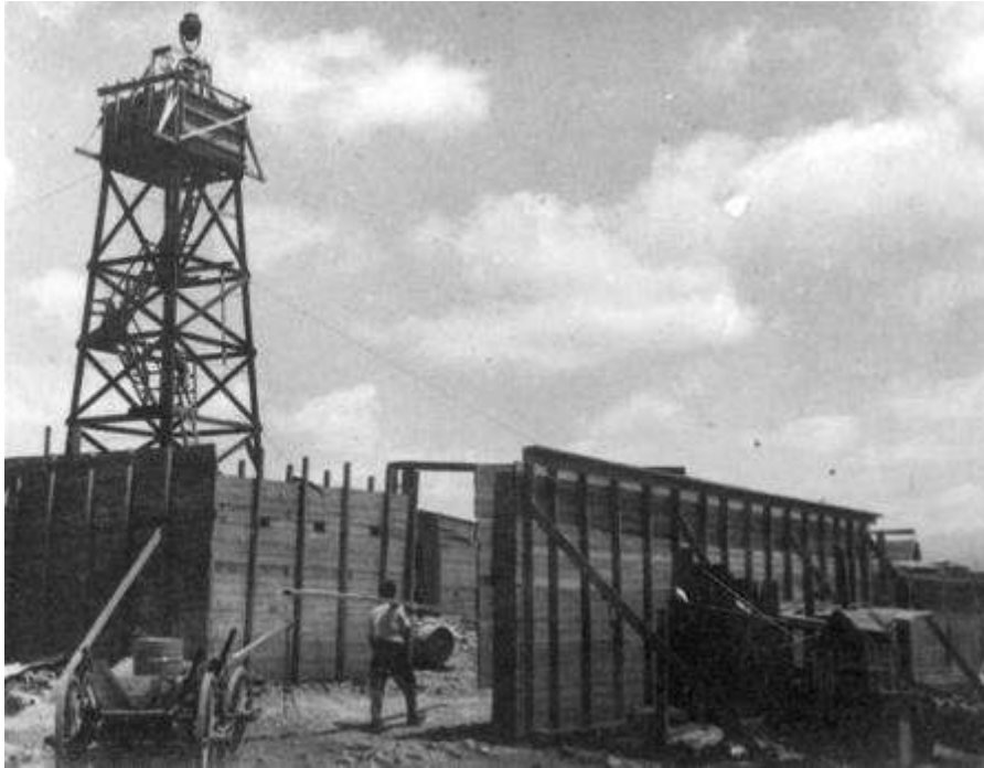
Building the Kibbutz Sha'ar HaGolan using Wall and Tower construction method, 1937. Source: PikiWiki – Israel free image collection project
